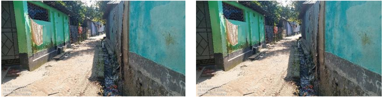
D-009: Construction of RCC Drain, starting from Rail Gate to Proposed Drain D-007 near h/o Mojibor Sangbadik (Ch 0.00m - Ch. 201.00m), at Ward no.- 5, Patgram Paurashava, Lalmonirhat. Total Length = 201m.
